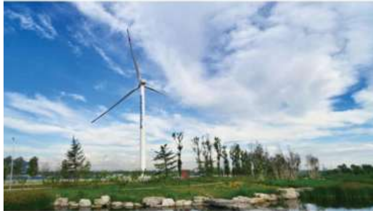
Industrial park low-carbon application
