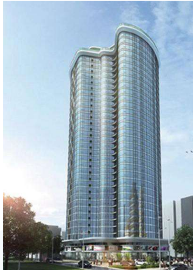
Office building-华地
